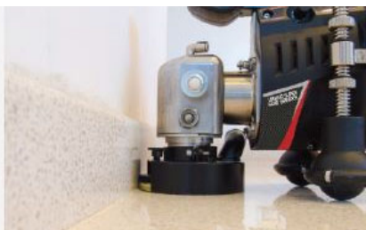
Grinding and polishing perimeters and edges.
