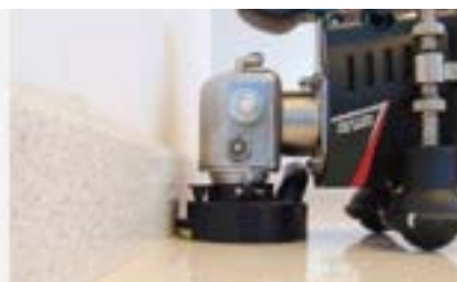
Grinding and polishing perimeters and edges.
